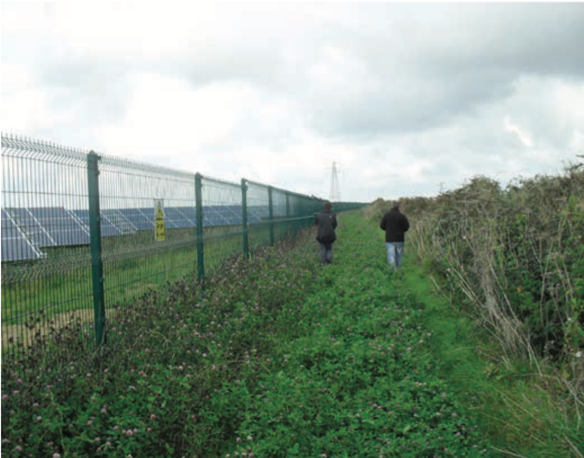
Photo showing security fence surrounding solar panels
