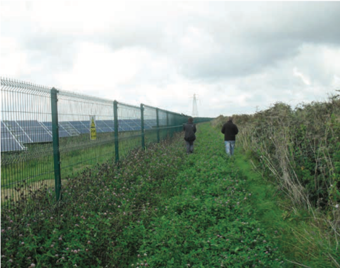
Photo of high security fencing surrounding a solar farm
